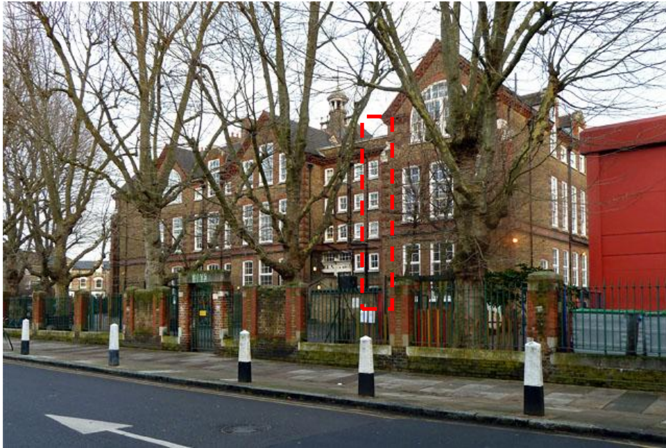
View from Perth Road Location of flue set behind decorative quoin detail
